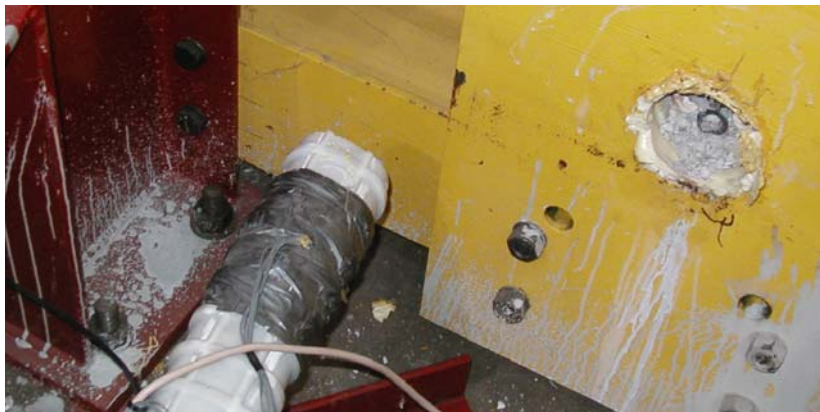
Figure 6-4 Fracture of all wires at north end of Specimen 1
