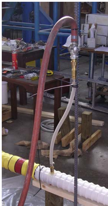
(a) Grout hose from pump
